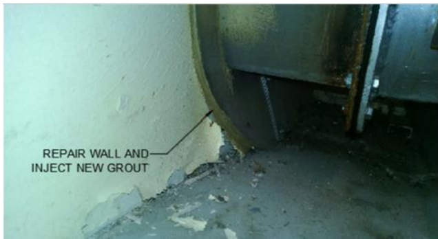
Damage done to the inside of the wall and pipe due to settlement at the east penetration, along with recommended reparations.
