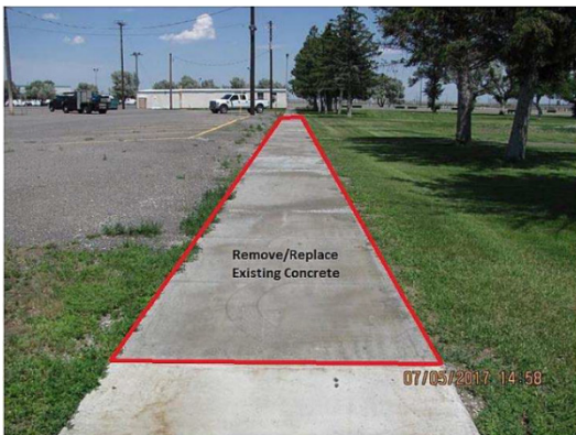
Figure 3. CFA-614 to CFA-685 Sidewalk Replacement
