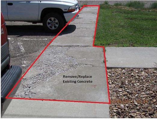
Figure 4. CFA-615 East Side Sidewalk Replacement
