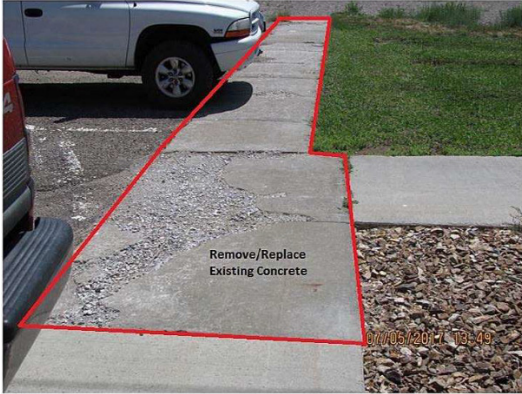
Figure 4. CFA-615 East Side Sidewalk Replacement
