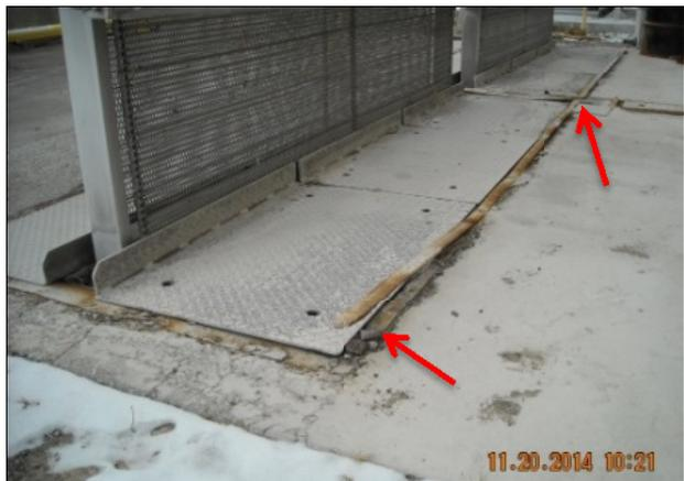
Figure 1. Proposed work metal strip removal.
