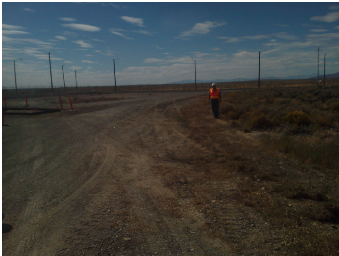
Figure 1. Interior perimeter road near TRA-680 proposed for widening.
