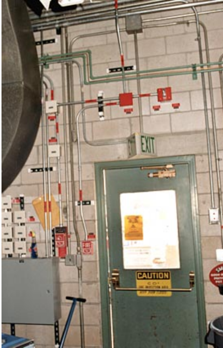
Figure 3-3. “Panic hardware” installed on TRA-648 emergency exits.
