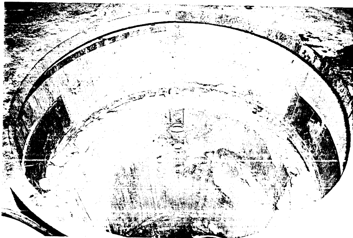
Figure II-25 Inside of Support Cylinder
