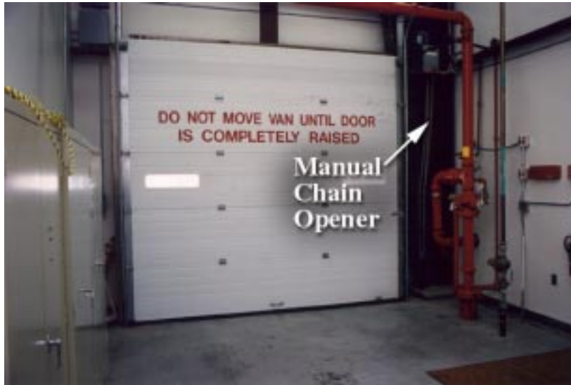
Exhibit 2-6. Emergency Control Center Door
