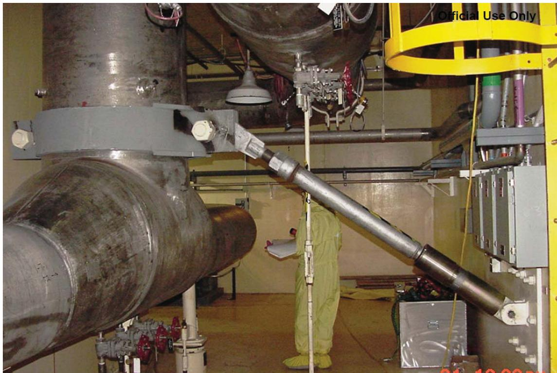
M1-1-7-N61-WSNG-DSC00105 (Used to determine length of clamp cantilever, connection, and anchorage location)
