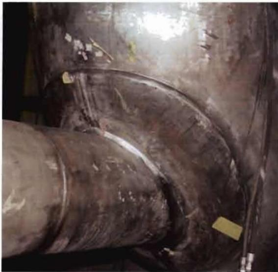
Pilot Model unlisted branch component => 14" branch extended from 36" elbow
