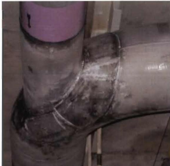
Model (256) unlisted branch component => 10" branch extended from 16" elbow
