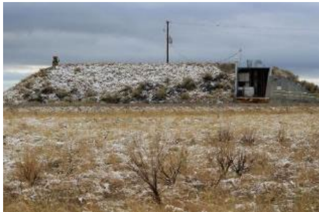
Figure 2. CF-638, northeast façade
