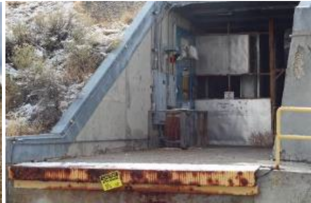
Figure 3. CF-638, entrance on southeast façade
