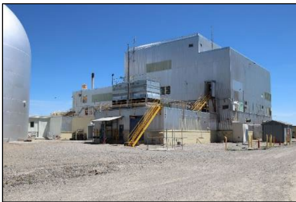
Figure 27. MFC-768, north and west façades (CEMML 2021)
