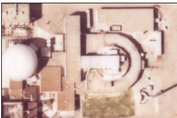
Figure 16. MFC-765 aerial imagery, 1982 (EG&G Idaho, Inc. 1982)
