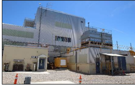
Figure 7. MFC-768, second and third sections of north façade (CEMML 2021)
