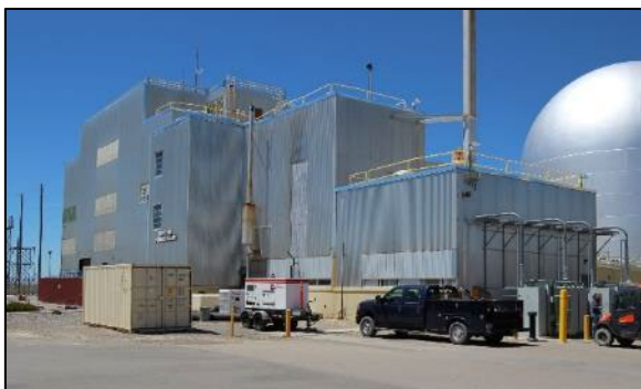
Figure 41. MFC-768, south and east façades (CEMML 2021)
