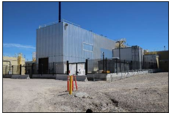
Figure 6. MFC-765, north and west façades (CEMML 2021)
