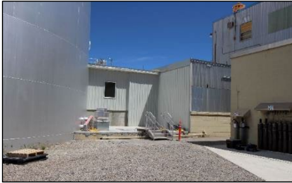
Figure 65. MFC-768, first section of north façade (CEMML 2021)
