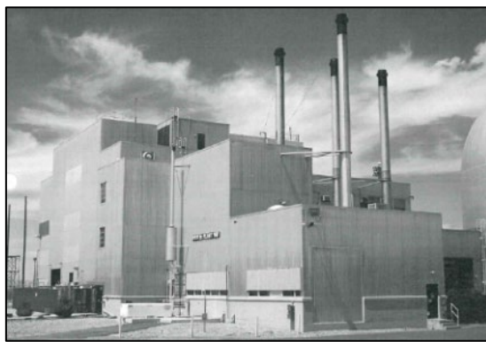
Figure 37. MFC-768, south and east façades, 2012 (Argonne National Laboratory No Date)
