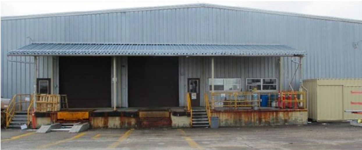
MFC-781 North End of Building
