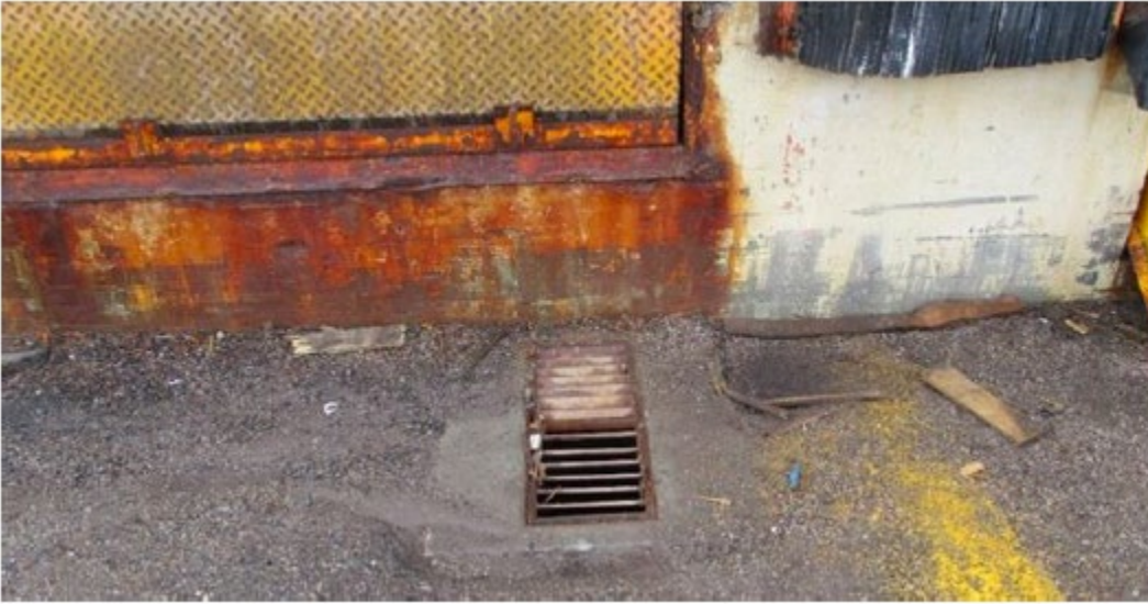
Drainage Inlet in Middle of Dock
