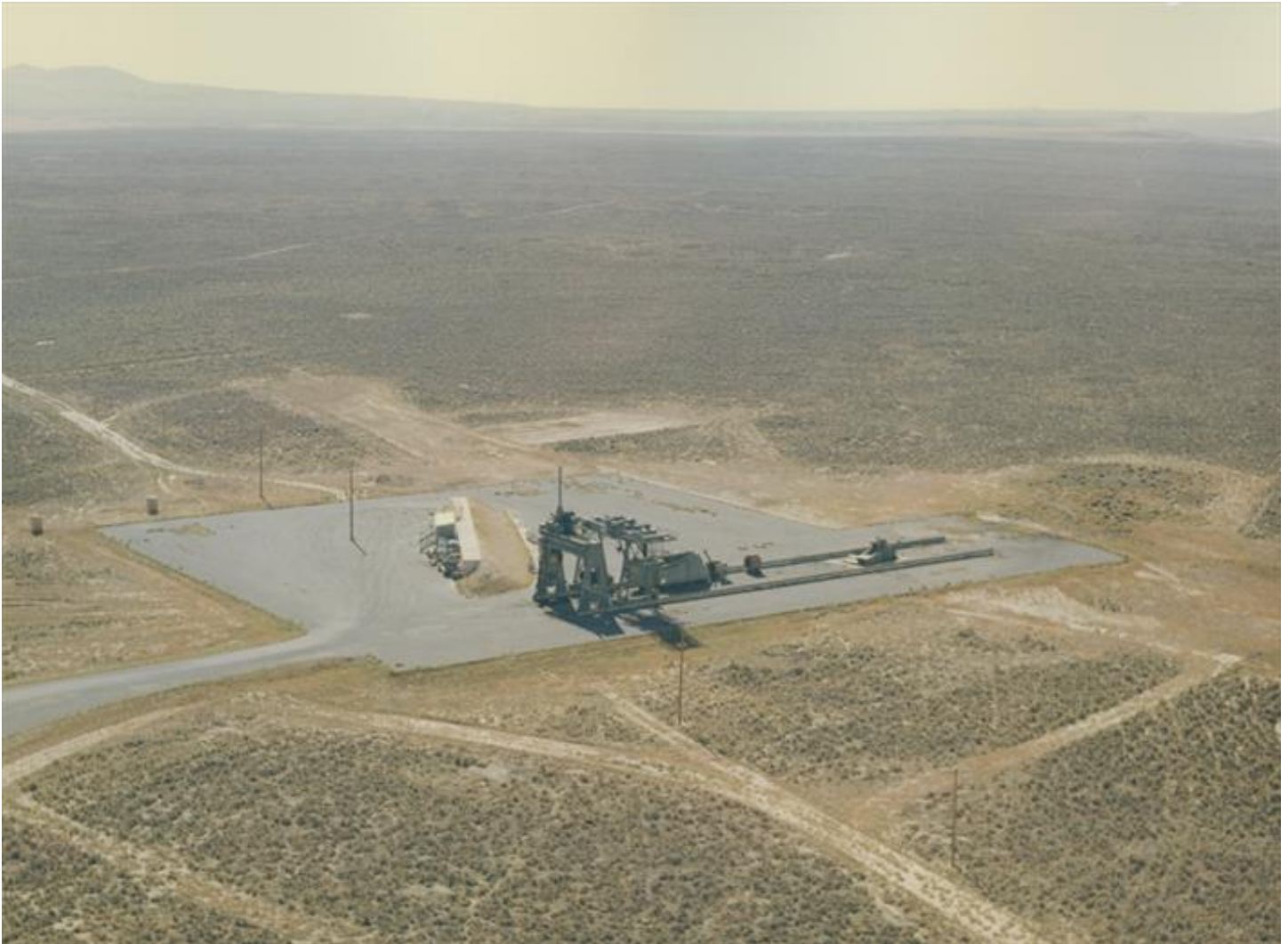
Site Current Conditions
