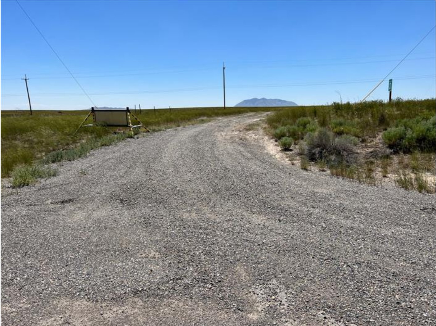
Photo 2: View of the road entrance to Pad D.
