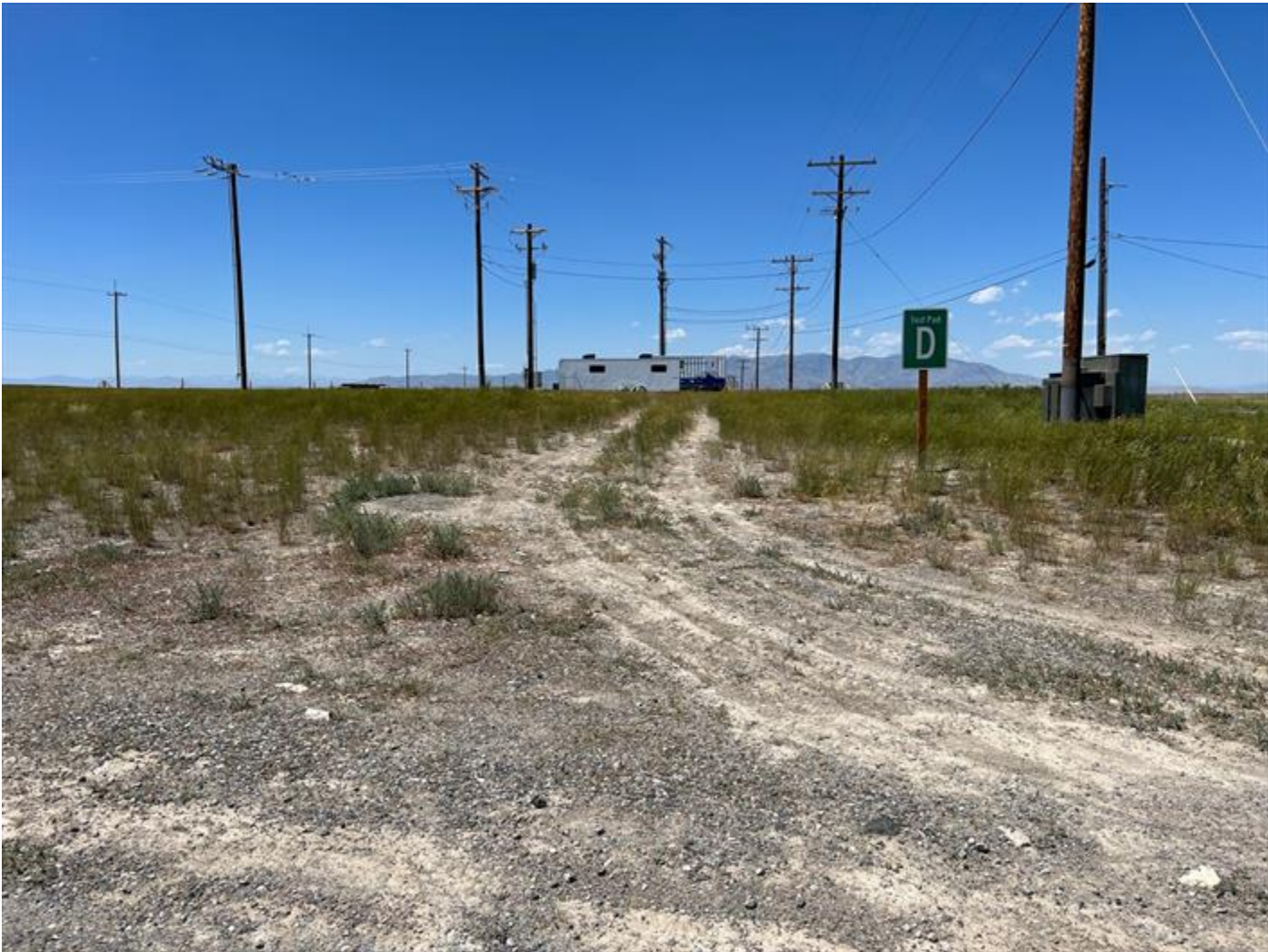
Photo 3: Current conditions of the two-track dirt road to Pad D.
