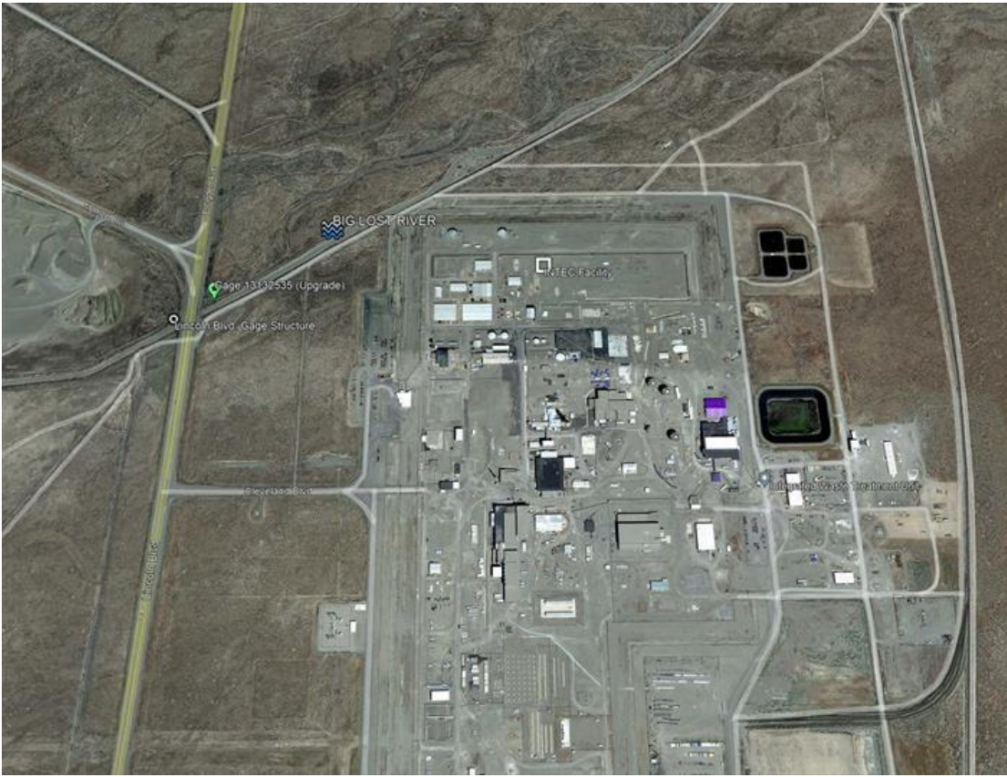
Figure 2. Gaging station location
