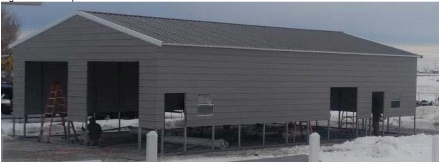
Figure 2-3: Example of the steel structure
