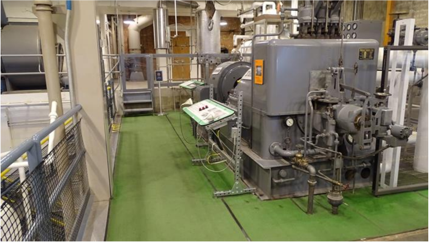
Figure 4. Green carpet in Turbine Area.
