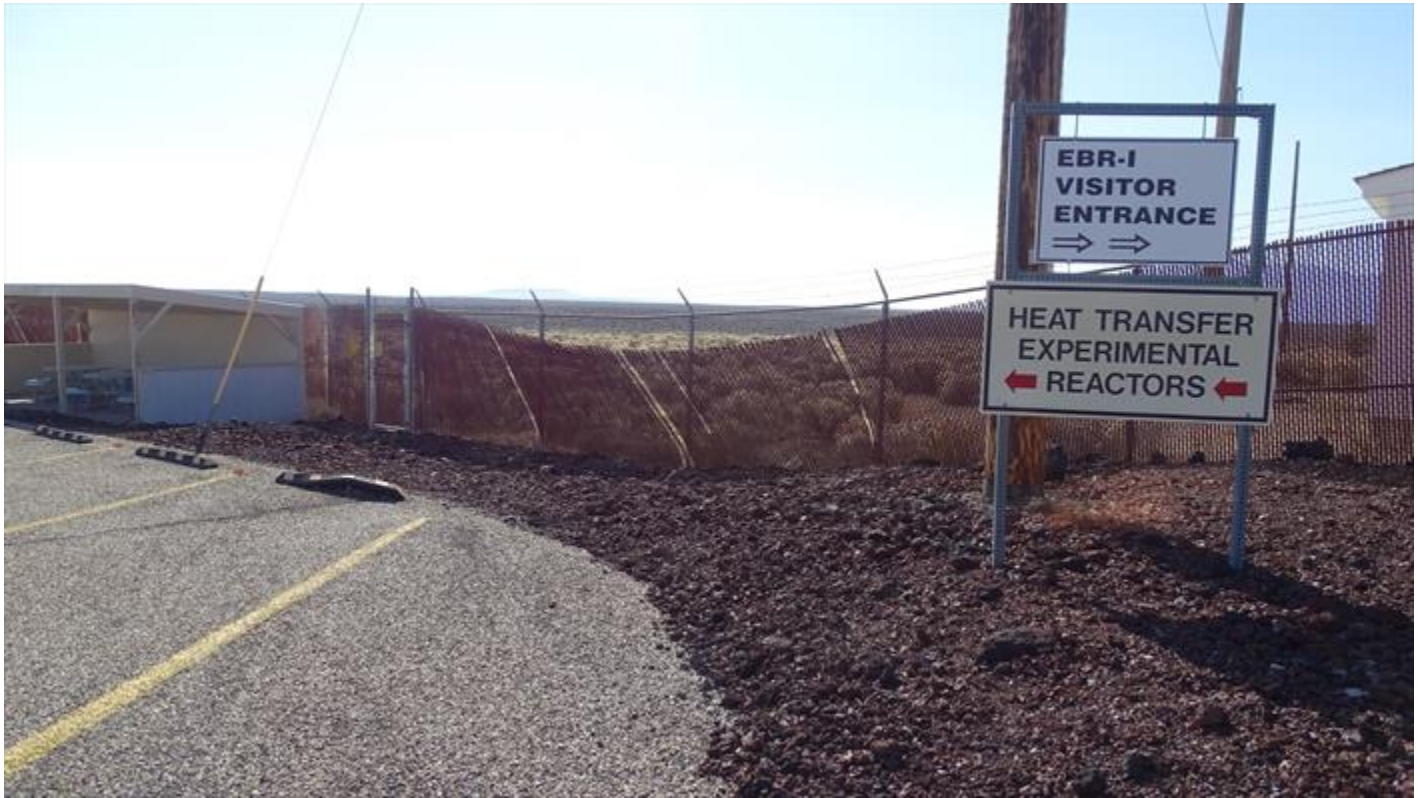
Figure 10. Current condition of fencing.
