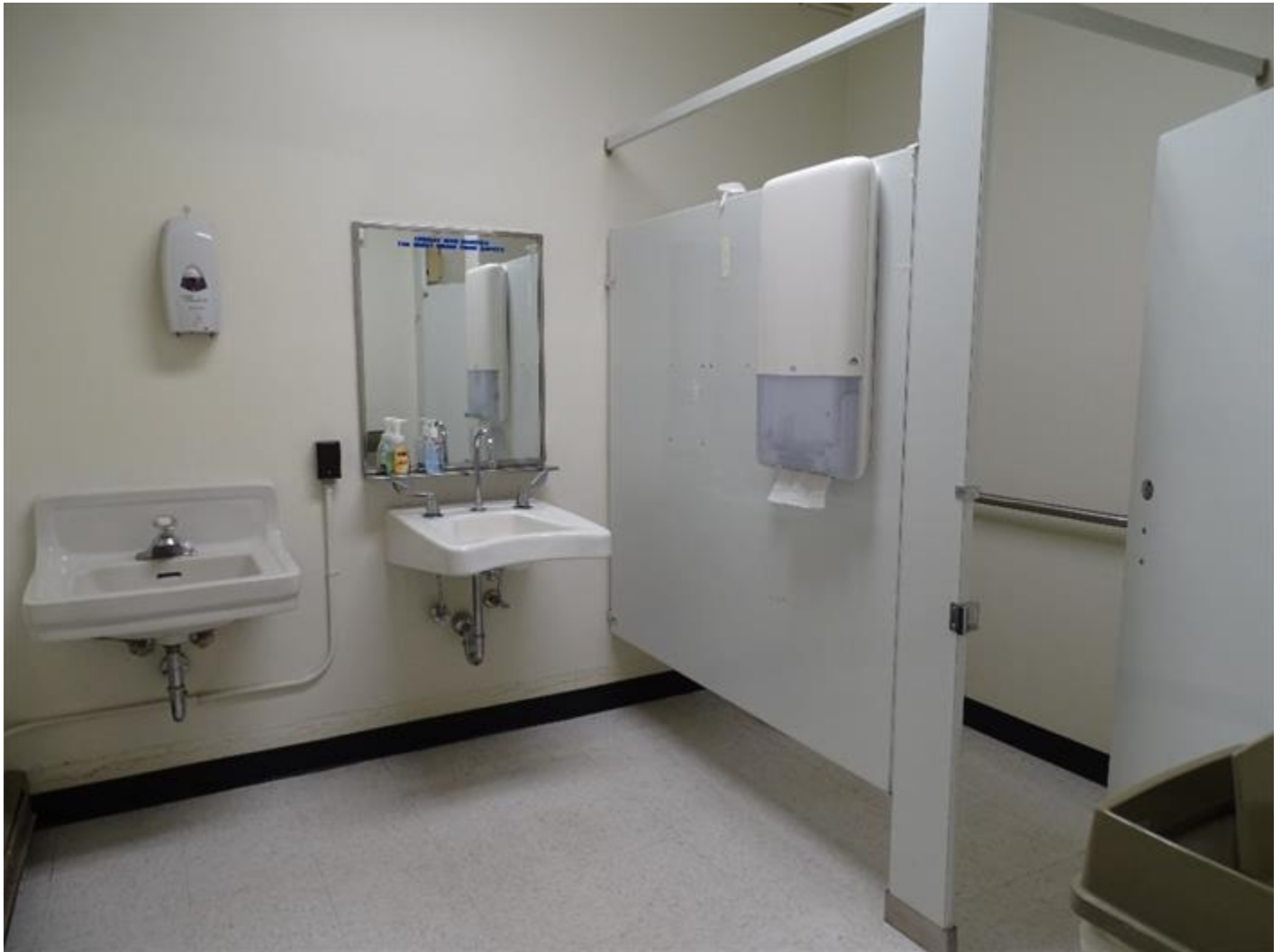
Figure 7. Annex Women's Restroom.
