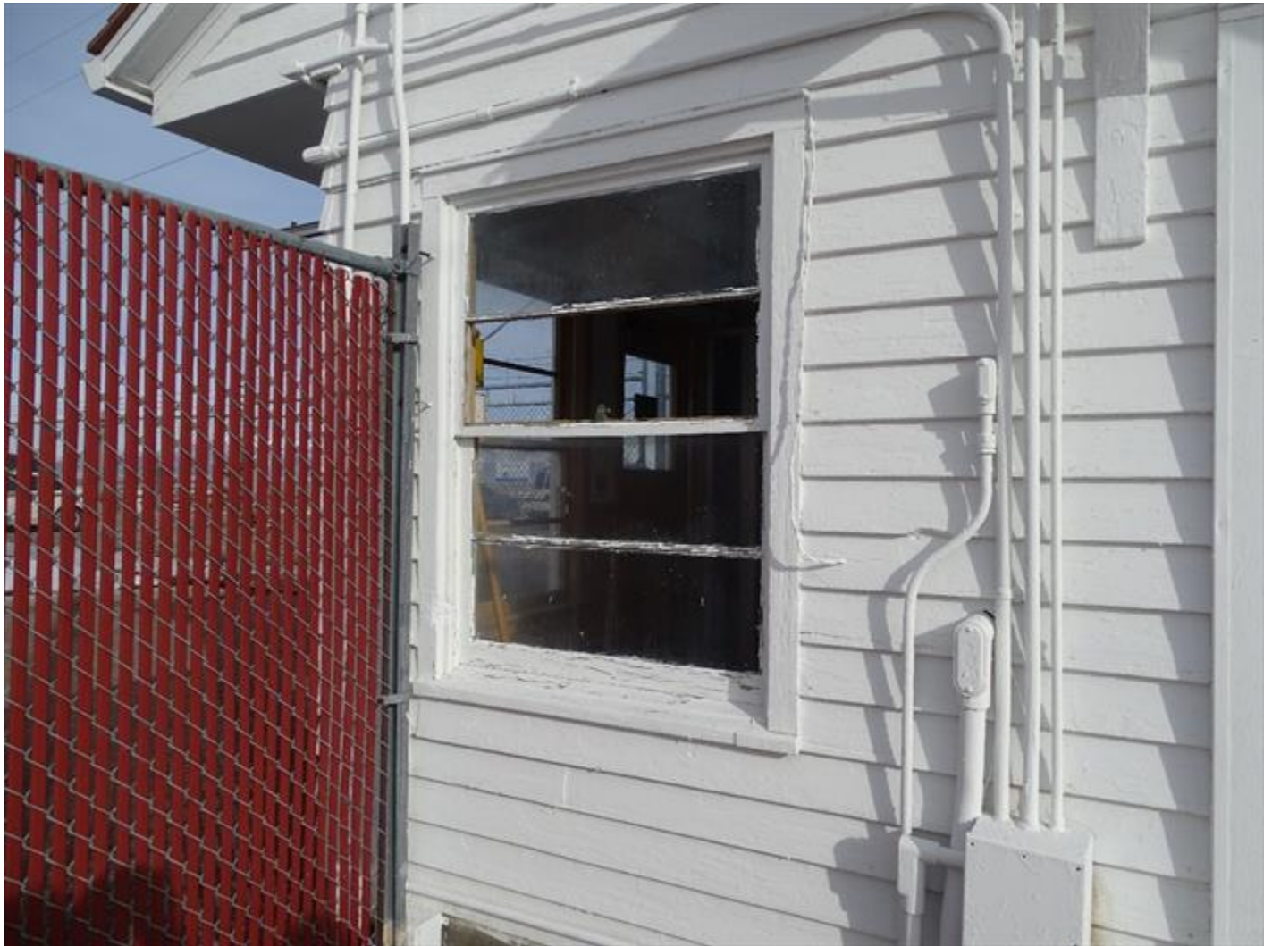
Figure 3. South window, EBR-I-602, showing failed glazing on lower pane of upper sash and generally poor condition of remaining glazing.
