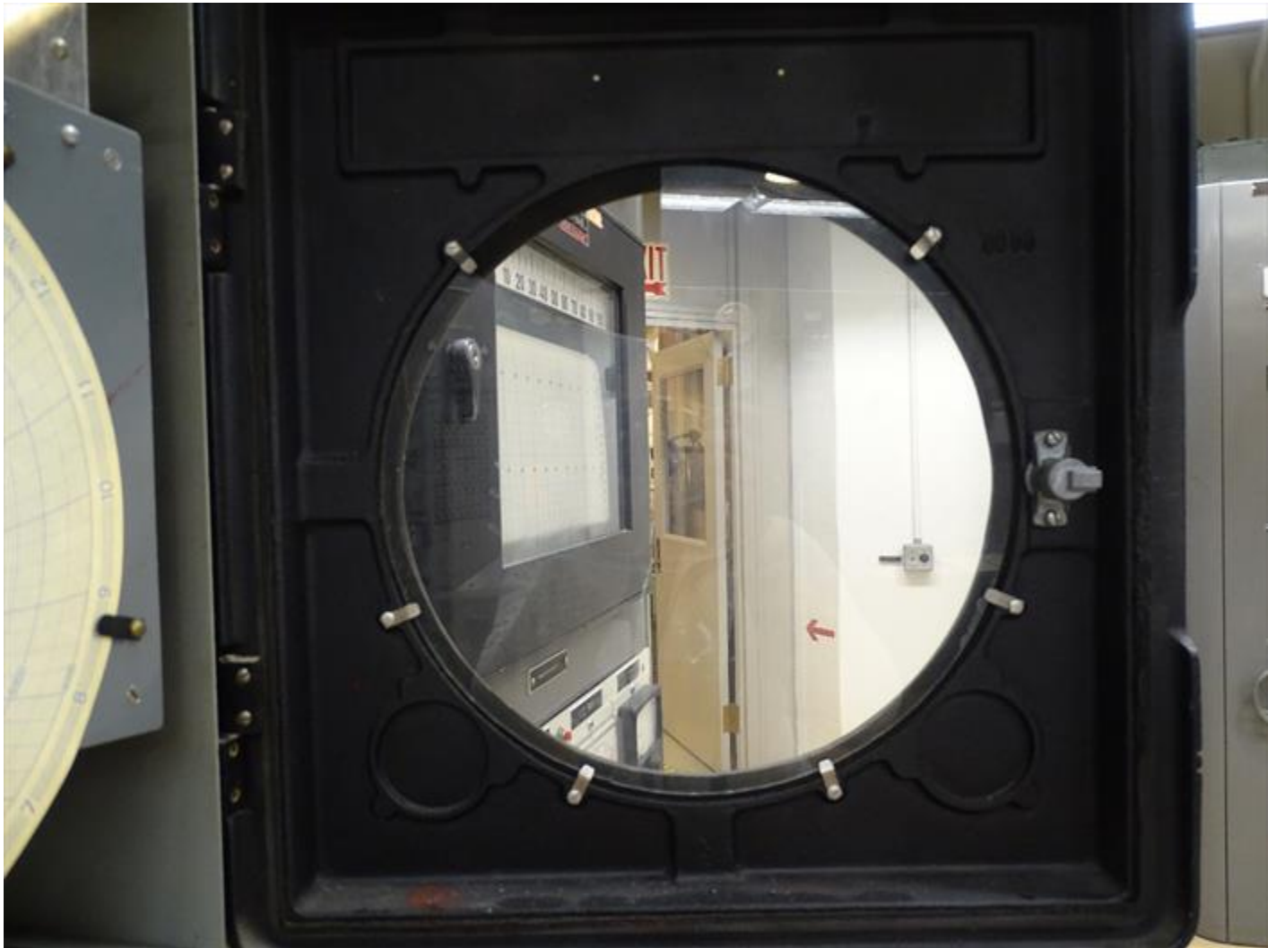
Figure 2. Broken glass face on EBR-I Control Panel, interior.
