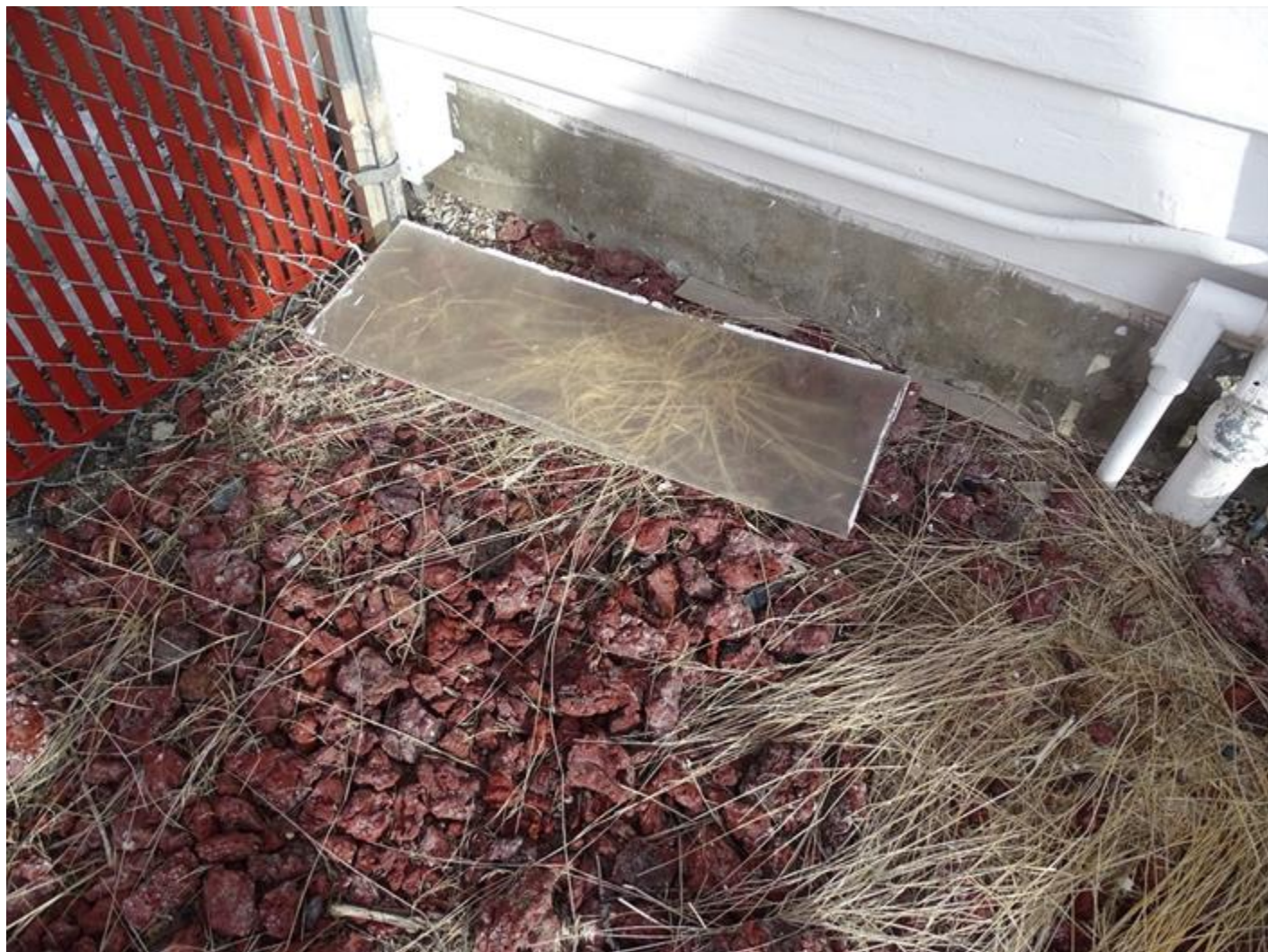
Figure 4. EBR-I-602, lower pane of upper sash appears to be a replacement using a non-glass substitute, such as acrylic or Lexan. Pane appears to be undamaged and suitable for reinstallation.
