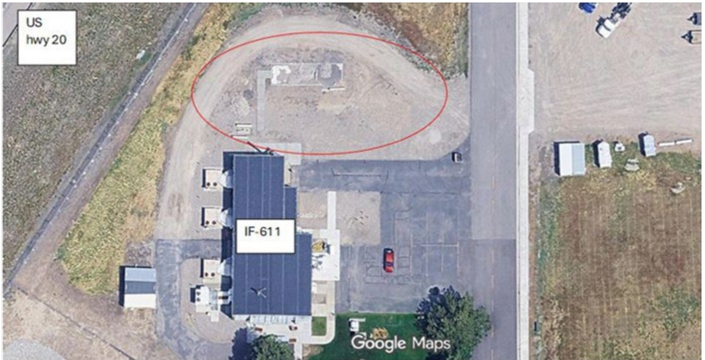
Figure 2: IF-611 possible location for Conex box (location A).
