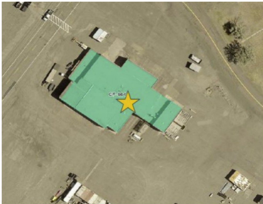
Figure 1. CF-664 Storage Building
