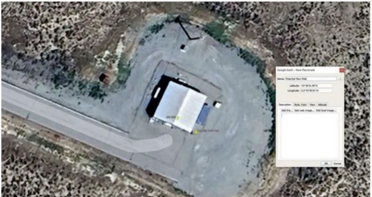
Figure 1, Rev. 2: B27-606 pole location.
