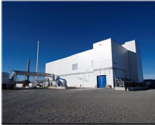
Integrated Waste Treatment Unit (IWTU)
