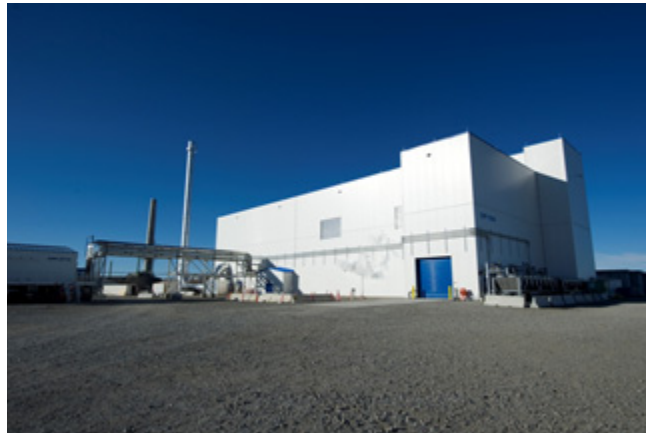
An exterior view of the Integrated Waste Treatment Unit
