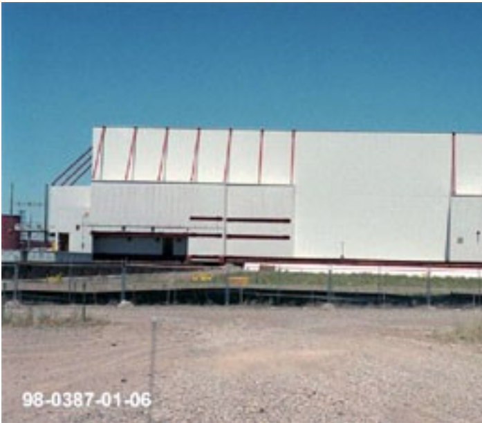
The original Pit 9 project included a retrieval building constructed on rails. It was designed to roll over the pit and remotely excavate buried waste. The retrieval facility was never used, and the contractor was ordered by the courts to pay for its removal.
