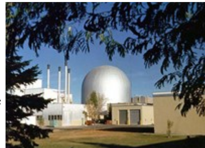
Experimental Breeder Reactor-II containment dome
