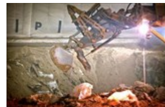
Waste exhumations continue at the Accelerated Retrieval Project.
