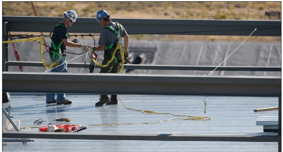
Two Idaho Cleanup Project workers install deck plate material on the mechanical building section of the IWTU.
