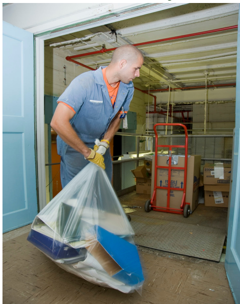
(Above) Workers remove legacy materials from Y-12’s Beta 4 facility. Material removal in this facility was 13% complete at the end of June.
