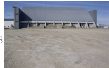
Loss-Of-Fluid Test Reactor Facility (after)
