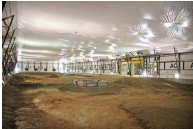
Inside the retrieval enclosure at Accelerated Retrieval Project-III
