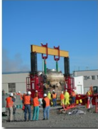
Gantry jacks attached to ETR vessel. Initial lift starts. - Click on image to enlarge.
