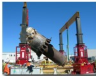
130 ton vessel positioning for transport. - Click on image to enlarge.
